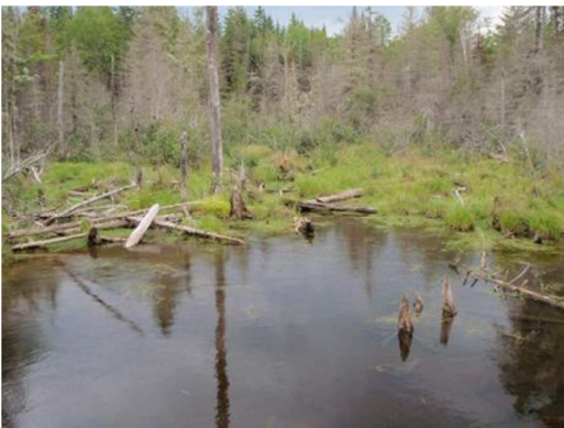
Water ponded upstream of an old crossing is a good indication that the crossing is set at too high an elevation
