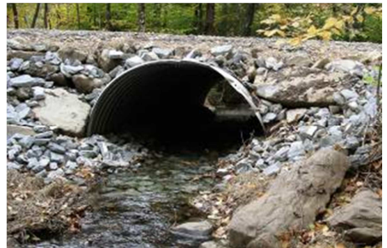
A culvert that is spanning the stream channel
