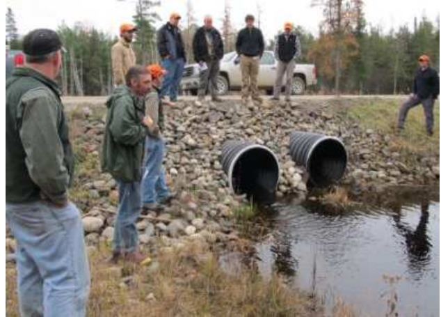
Field training session on culvert installation
