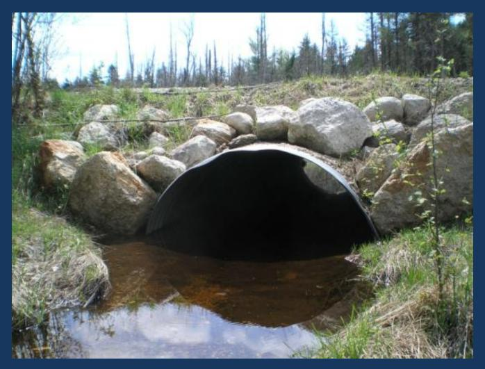
8' span 40' long ~\$6,800 installed
