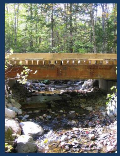
22' span bridge \$6,200 Materials - \$11,200 Installed
