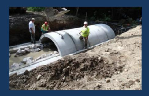
8' span 40' long ~\$9,600 installed
