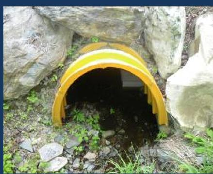
3.5' span 32' long \$2,800 installed
