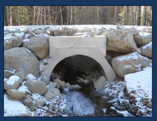
5' span 32' long ~\$3,000 installed
