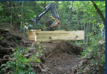
To' long 10' span under 8' of fill ~\$10,000 installed
