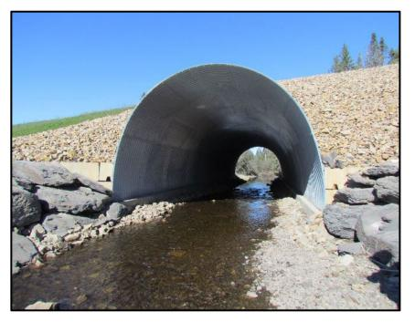
Preferred methods of restoring fish passage at problem sites would include bridges, arches, embedded and total removal.
