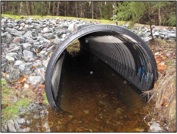
Round pipes, properly installed, should not be disregarded when considering options for fish passage improvement.
